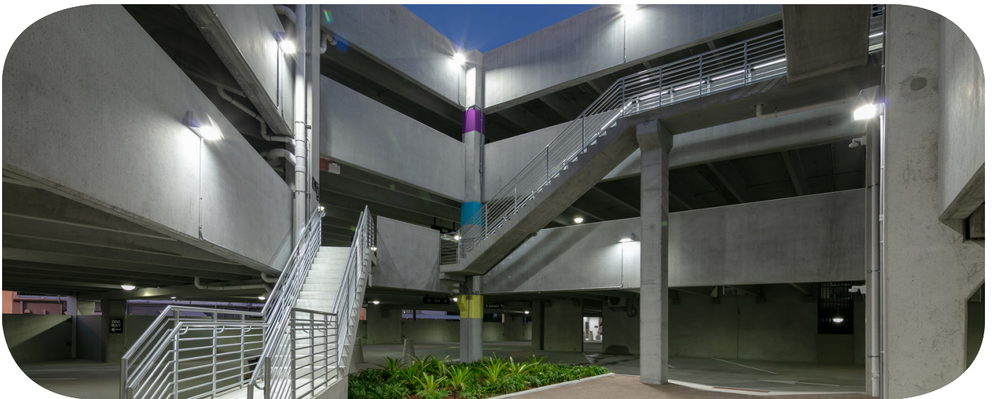
Photos Courtesy of Jon F. Swift Construction
